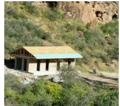
The WB Stowe Showerhouse and Restroom Facility now has a roof
