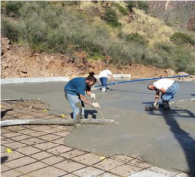
Workers smooth the concrete foundation
